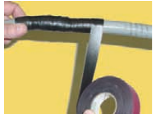
Tape will create a sealed protective covering
